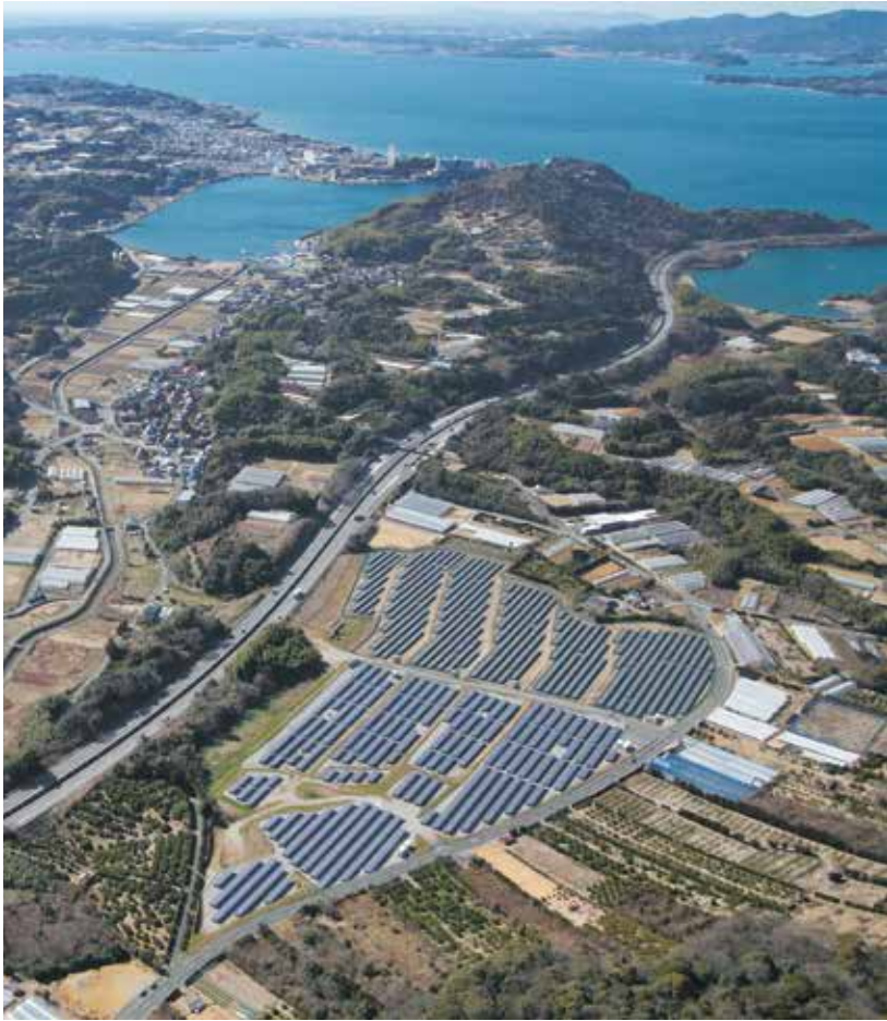
Solar Panels near Lake Hamana
